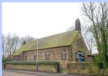
St. John's Backworth
