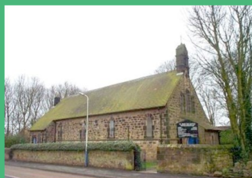
St. John's Backworth
