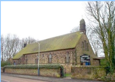
St. John's Backworth
