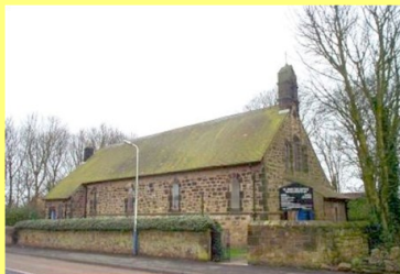
St. John's Backworth
