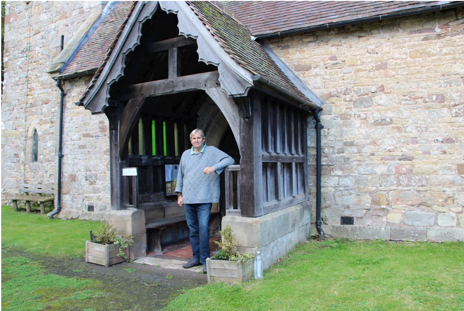
The wooden porch at St John the Baptist, Nash.
