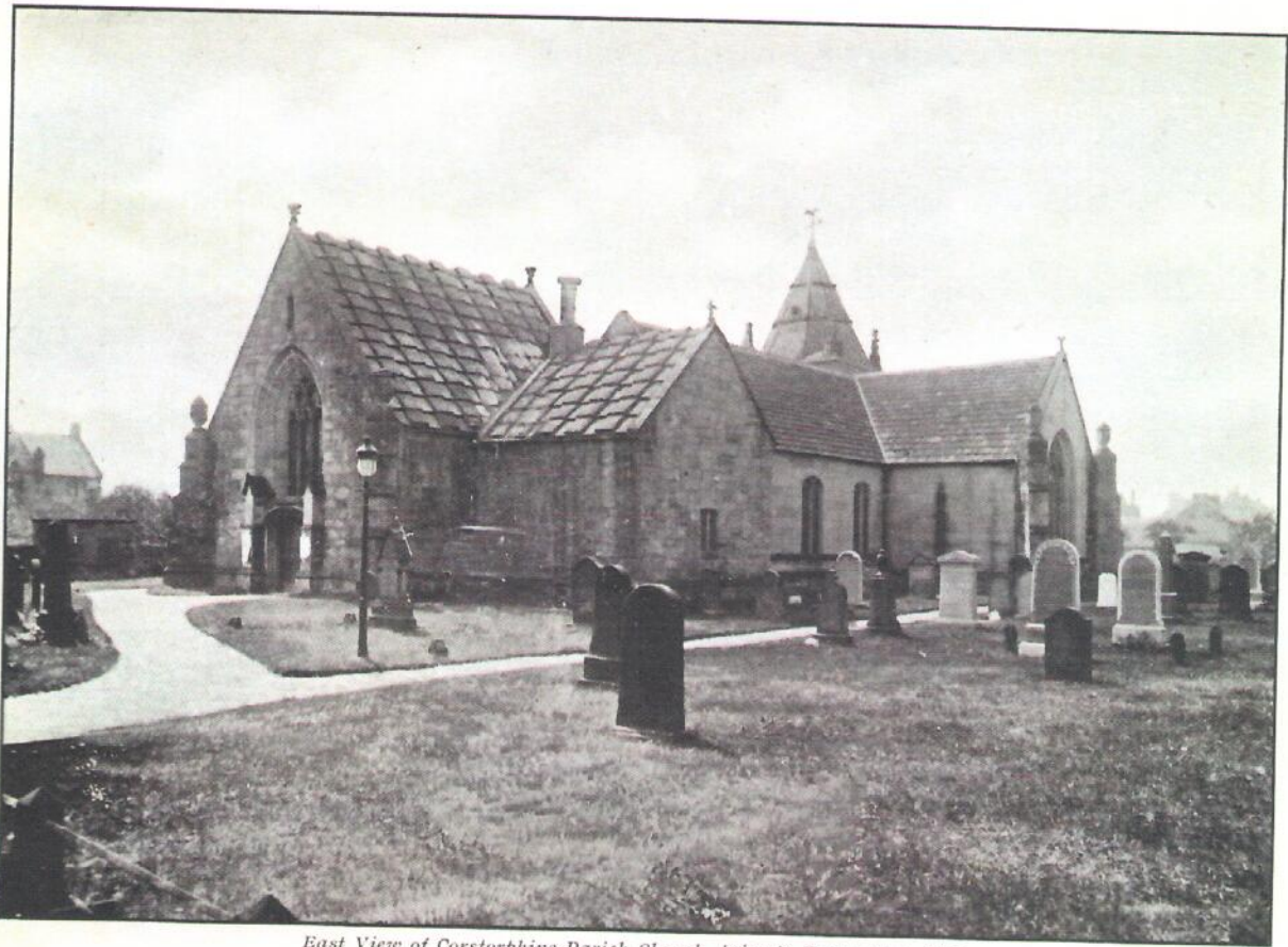
East View of Corstorphine Parish Church, prior to Restoration, 1905.
