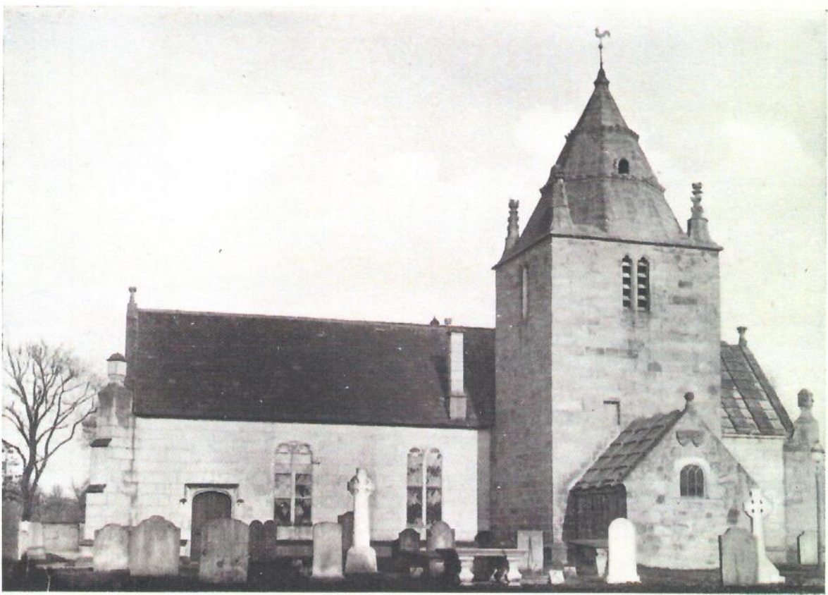
West View of Corstorphine Parish Church, prior to Restoration, 1905.
