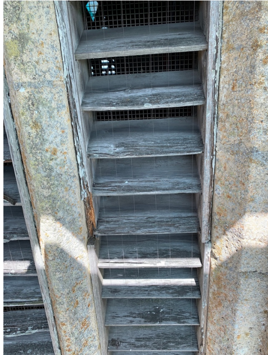
Poor condition of louvres on S face -will be replaced from inside the tower
