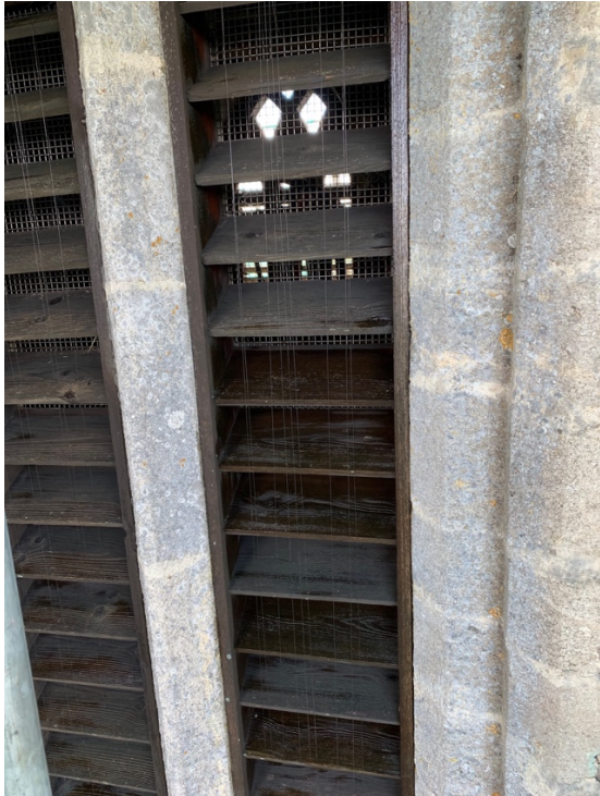
Treated louvres on N face – good condition
