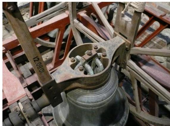
Fig. 8. Canons, iron straps and wooden headstock and a steel canon-retaining headstock
