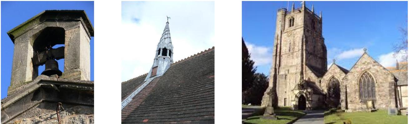
Fig. 2. A stone turret above a gable end, a flèche midway along a roof apex and a massive masonry tower
