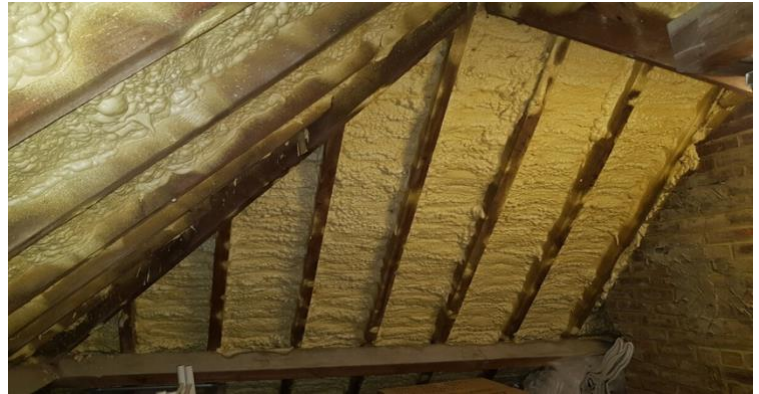
Figure 8 – Example of spray foam insulation in a roof
