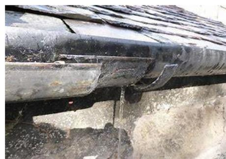
*Figure 3 – Example of a leaking gutter*
