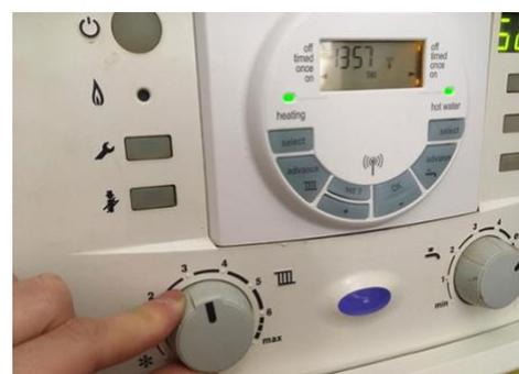
Figure 7 - Example of a person adjusting the **boiler flow temperature**
