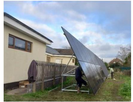
*Figure 14 – Ground-mounted Solar PV array at one of our churches.*
