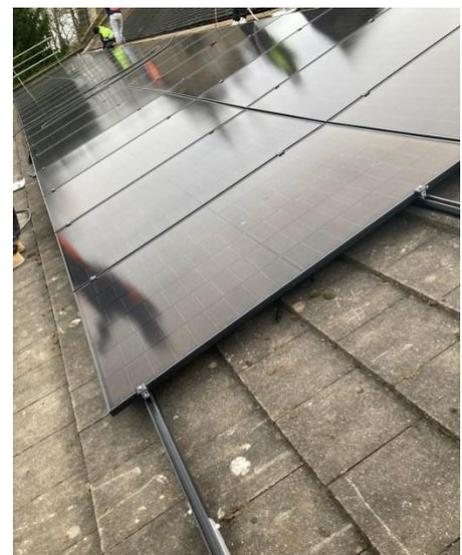
*Figure 13 – Roof-mounted Solar PV array on one of our churches.*
