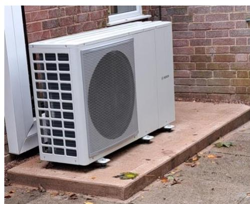
*Figure 9 – An air-source heat pump in-situ at a Vicarage in our Diocese.*
