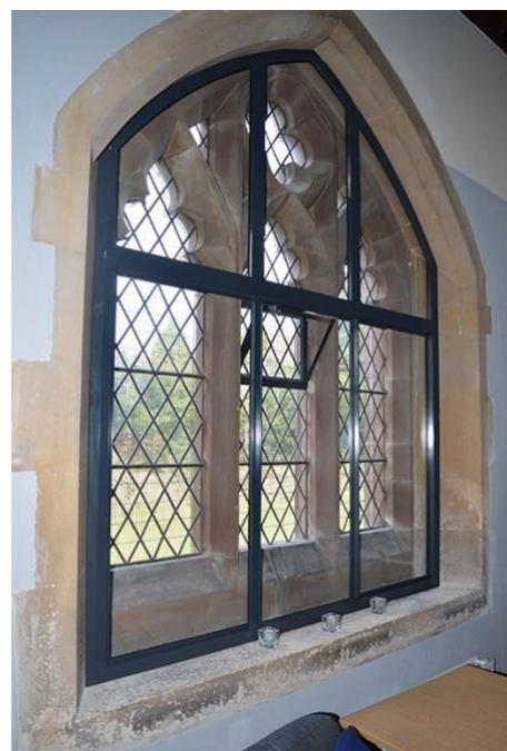
*Figure 6 – Example of secondary glazing in a church.*
