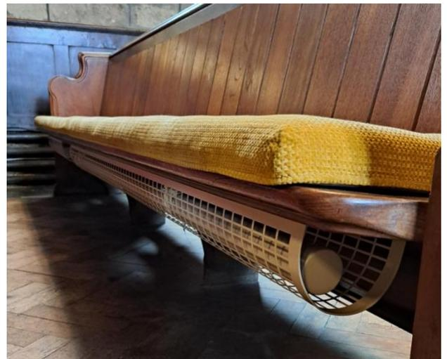
*Figure 10 – Example of under-pew heaters in-situ at one of our churches.*
