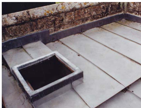
Lead used for flashings and access hatch capping
