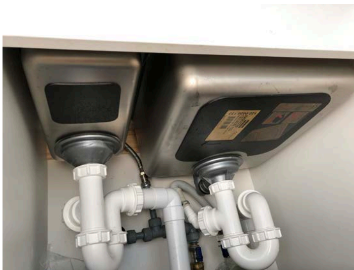
Mats bonded to underside of sink to reduce dripping noises
