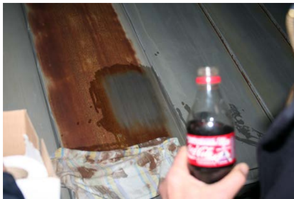
Stain successfully removed using weak phosphoric acid solution
