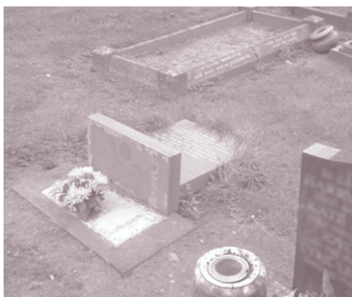
Inadequately secured memorial
