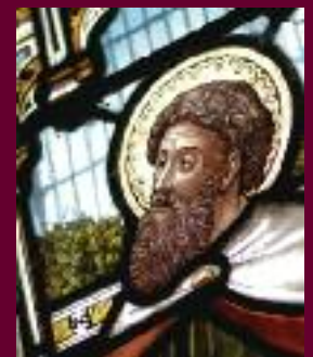
Stained glass windows, particularly those of historic interest, should be suitably protected against accidental damage.
