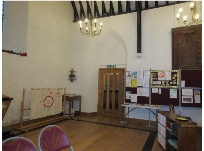
New internal entrance via porch
