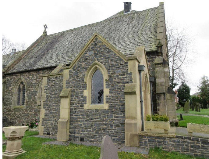
Porch design sympathetic to the historic building
