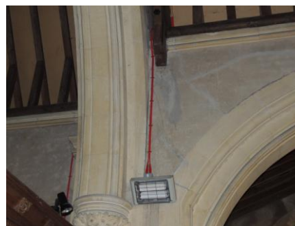
The choice of cable, colour and wiring runs may have a dramatic effect on the appearance of a church
