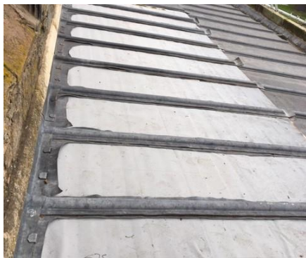
Lead cut away between the wood rolls
