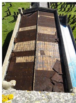
Nave Copper Roof completely stripped Temporary covering to aisle roof
