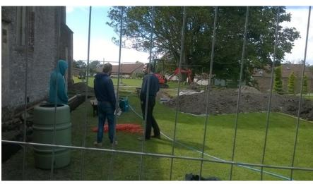
the past two months and are near completion. Ditches have been dug around the perimeter of the building with drainage pipes Inserted leading to a large soakaway in the middle of the graveyard, (behind the earth pile.) This work is to drain moisture away from the walls which inside are constantly damp and flaky.
