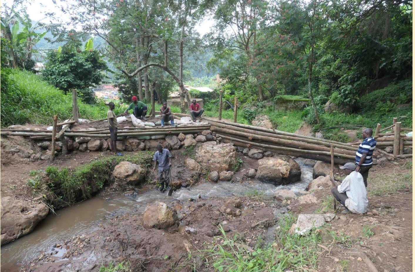
We have also opened up part of the main river channel where there was a bottle-neck near the generator house and put a protective wall around this to minimise the chance of damage.
