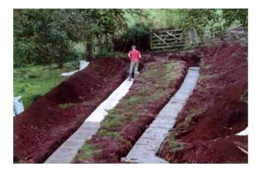
Figure 2. The trenches are now both covered by the slabs and the geotextile is laid on the top.
