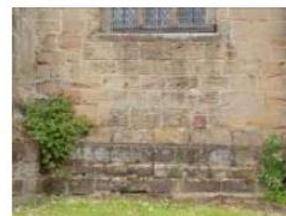
The north elevation, above the Choir Vestry roof, has failing cement overpointing leaving sound lime pointing behind. Stonework in fair condition with minor damage
