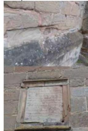
5.7 Priest's Vestry – The east gable stonework and pointing in fair condition with some individual stones weathered, some open jointing and moss/vegetation at plinth level. As elsewhere, cement pointing is aggravating damp and deterioration. The stone tracery of the window appears sound.
