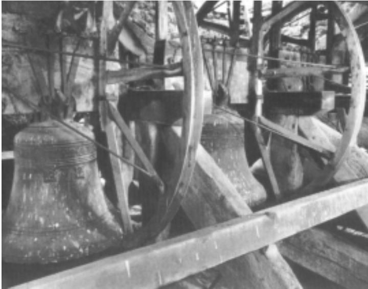
fig. 6 Short-headed queenpost frame (All Saints' Church, Knipton, Leicestershire)
