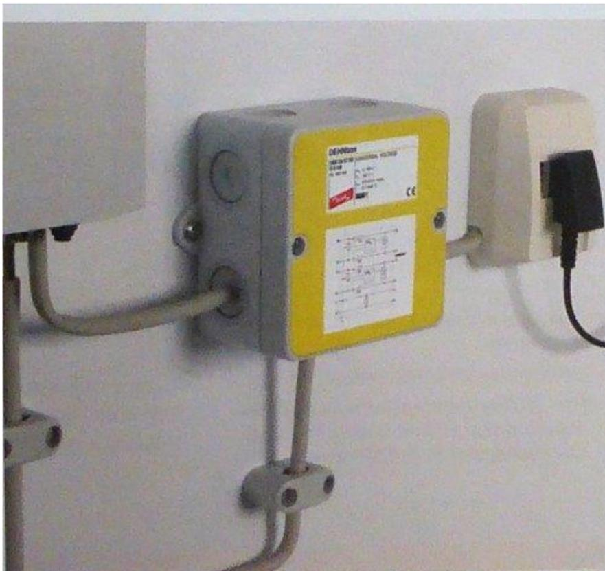
4. Dehn Type 2. As listed in Appendix 4, Dehn Surge protector DLI TC BT part number 929 026 is a generally suitable Type 2 plug-in device for a single BT in-use line to deal with the let-through surges from a Type 1 device.
