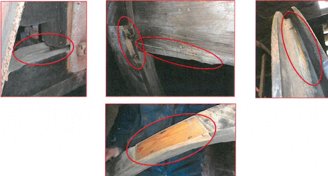
*Above: Images showing the condition of the bell wheels, including: Split spokes, burst feather fillets, replacement shrouding, and worn soling.*
