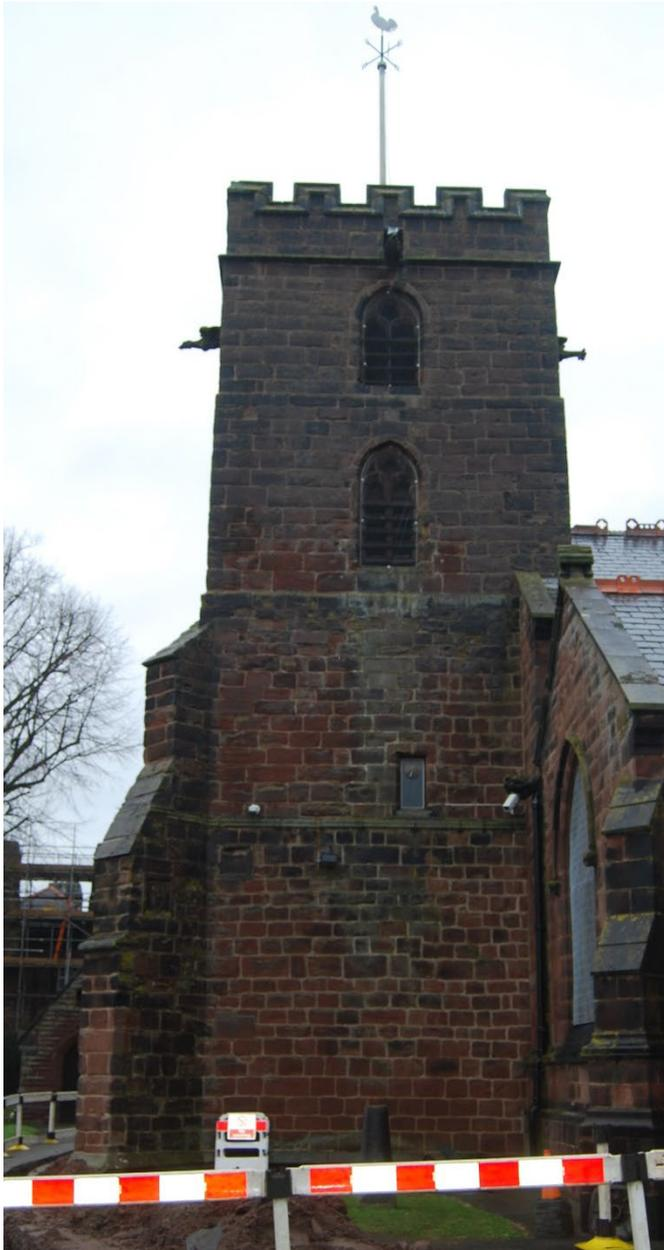
This wall contains louvre window openings at belfry and clock chamber levels and a small, glazed window opening giving light to the ringing chamber. The masonry appears to be in generally fair condition, consistent with its age, with no evidence of any significant cracking, recent or ongoing movement.
