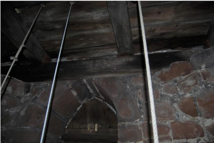
The walls at this level are of exposed stone masonry construction. There are what appear to be the beginnings of squinch arches below belfry floor level, the purposes of which are unknown. Possibly there was some intention of building a spire at some time in the past. There does not appear to be any evidence of significant cracking, recent or ongoing movement to the masonry.
