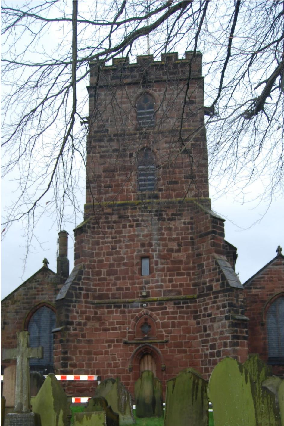
This wall contains louvre window openings at belfry and clock chamber levels, a small, glazed window opening giving light to the ringing chamber and a door opening at ground level with a small quatrefoil window immediately above this. Again, the masonry appears to be in generally fair condition, consistent with its age, with no evidence of any significant cracking, recent or ongoing movement.
