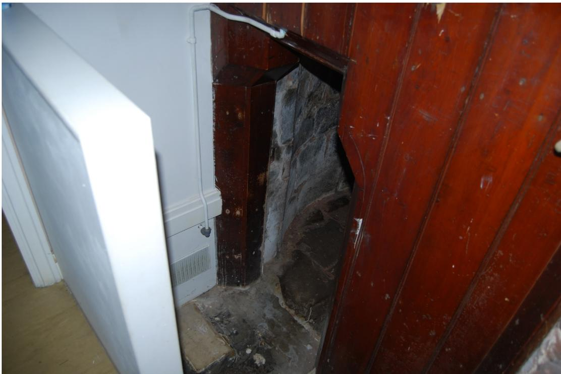
The original floor level has been raised to match the nave floor level. Toilets and a central heating boiler have been installed relatively recently. The walls, where exposed, have been painted and the masonry appears to be in generally fair condition, consistent with their age, with no evidence of any significant cracking, recent or ongoing movement.
