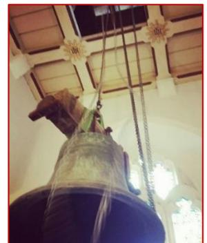
The Clock Hammer to be removed for overhaul and service.
