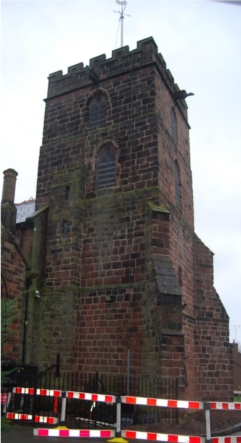
This wall contains louvre window openings at belfry and clock chamber levels. To the north east corner, there is a small projection which houses the spiral staircase and extends up to clock chamber level. There are two small window openings towards the top of this projection which give light to the staircase. Again, the masonry appears to be in generally fair condition, consistent with its age, with no evidence of any significant cracking, recent or ongoing movement.
