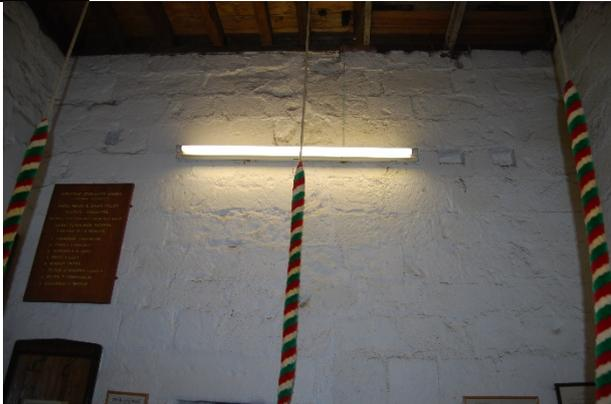
The walls at this level are partially obscured by timber panelling. Where they are exposed, they have been painted. There does not appear to be evidence of any significant cracking, recent or ongoing movement to the masonry.
