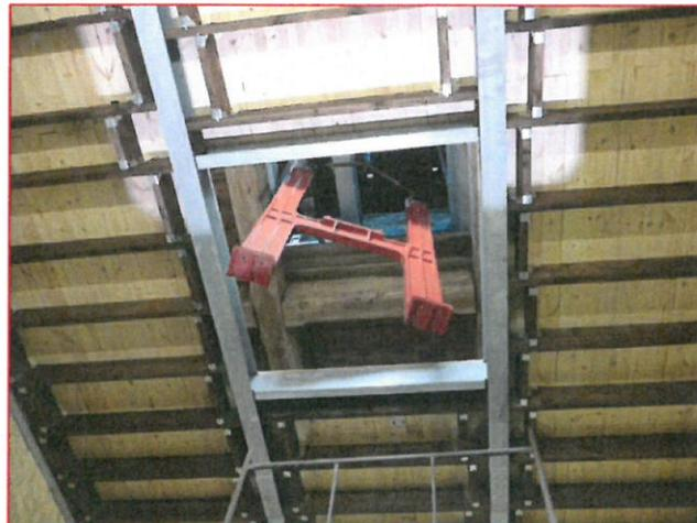
*Above: An image of a 'H' frameside passing through a floor that our bellhangers have recently built.*
