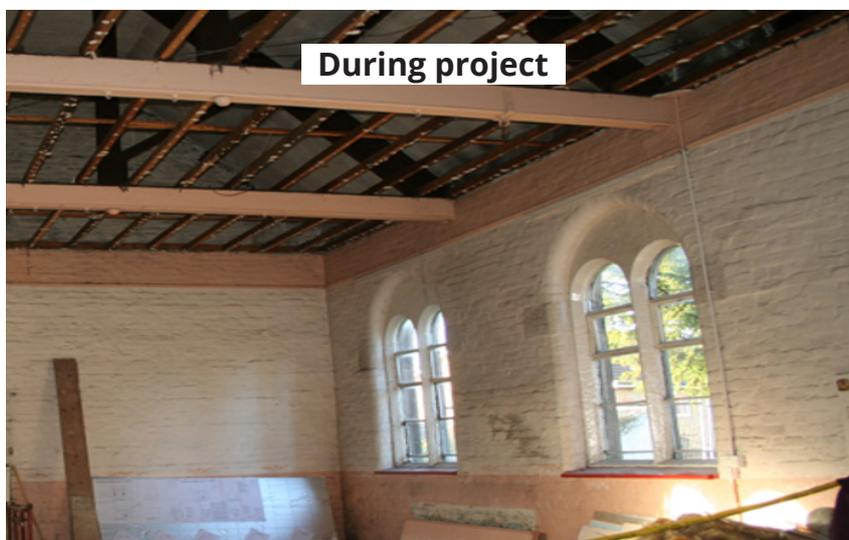
We first needed to make our church hall structurally sound. The 150-year-old iron nails were barely holding the roof slates in place, so it was a relief to find that most slates were in good condition. A vapour barrier (the Victorians didn't have such materials) was fitted and the slates refitted with copper galvanised nails. Cast steel guttering and down-spouts finished off the roof. Stone masonry was re-pointed, and all the old windows were replaced with heritage glazed units.
