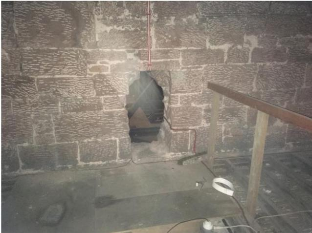
The main roof space (below) is directly connected to, and open to the tower, which has open louvres on four sides, ensuring constant and significant ventilation in the whole roof space.
