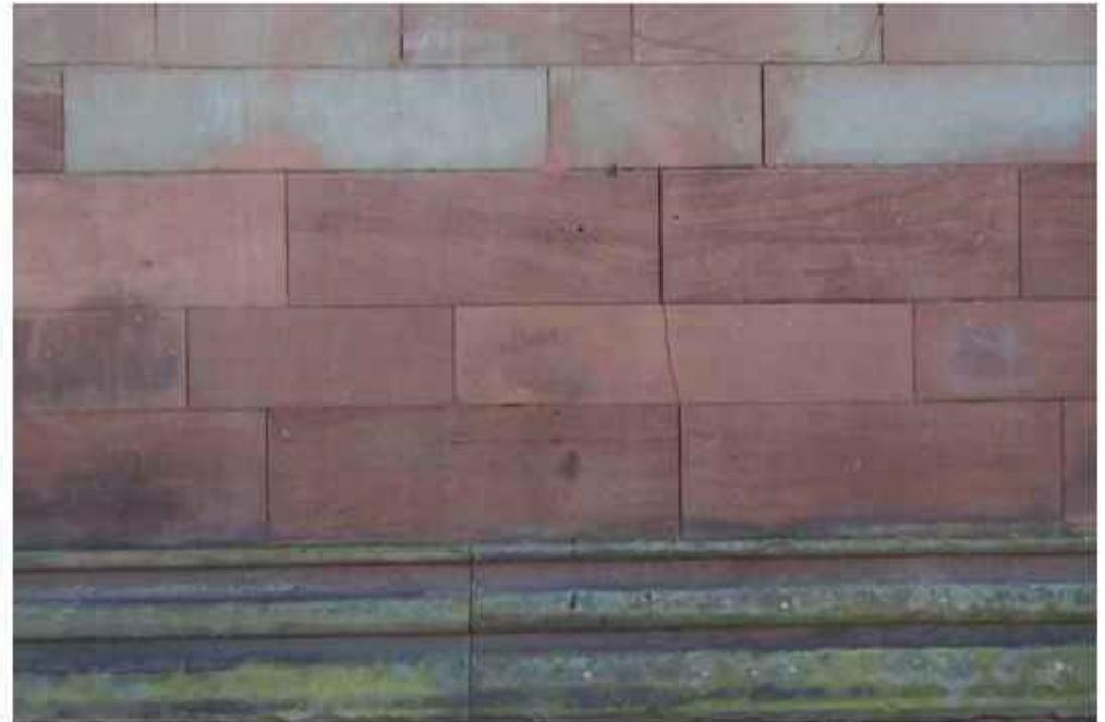
Images of stepped cracks below east window
