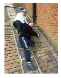
Dion Chapman and his son Dan set to work on the Western aisle lower roof essential repairs to the flashing and replacement to some of the damaged and crumbling tiles as pictured.
