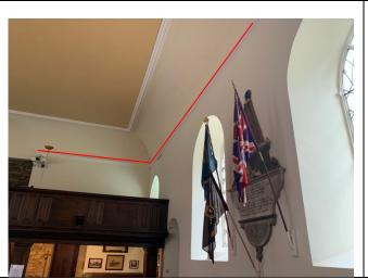
CAT6 cable from projector. Fitted in 25 x 16mm white trunking on top of picture rail.
