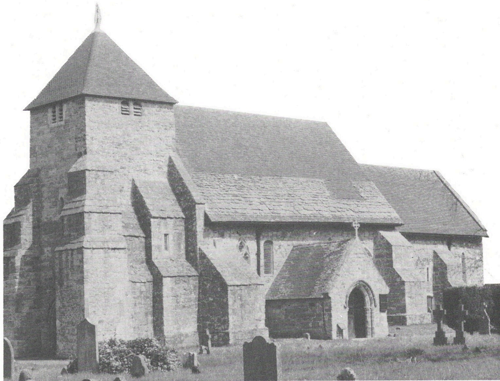
The last of the old stone roof tiles
