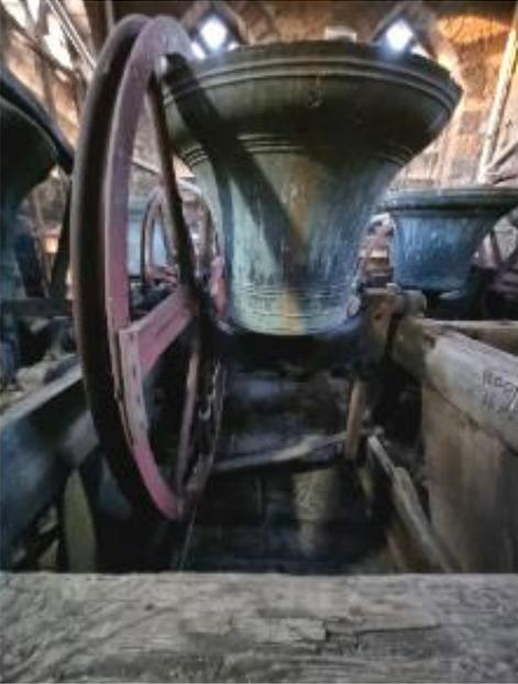
*Wheels and fittings, in a poor and worn out state*
