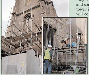
repair was clearly a priority and this will go ahead from 19th August for approximately two months. The work needs scaffolding, so that it can be done safely and this will go up outside of the tower. At the same time a lightning conductor is being installed and some masonry at the top of the tower is being stabilised. The work will cost over £57,000 and is being
