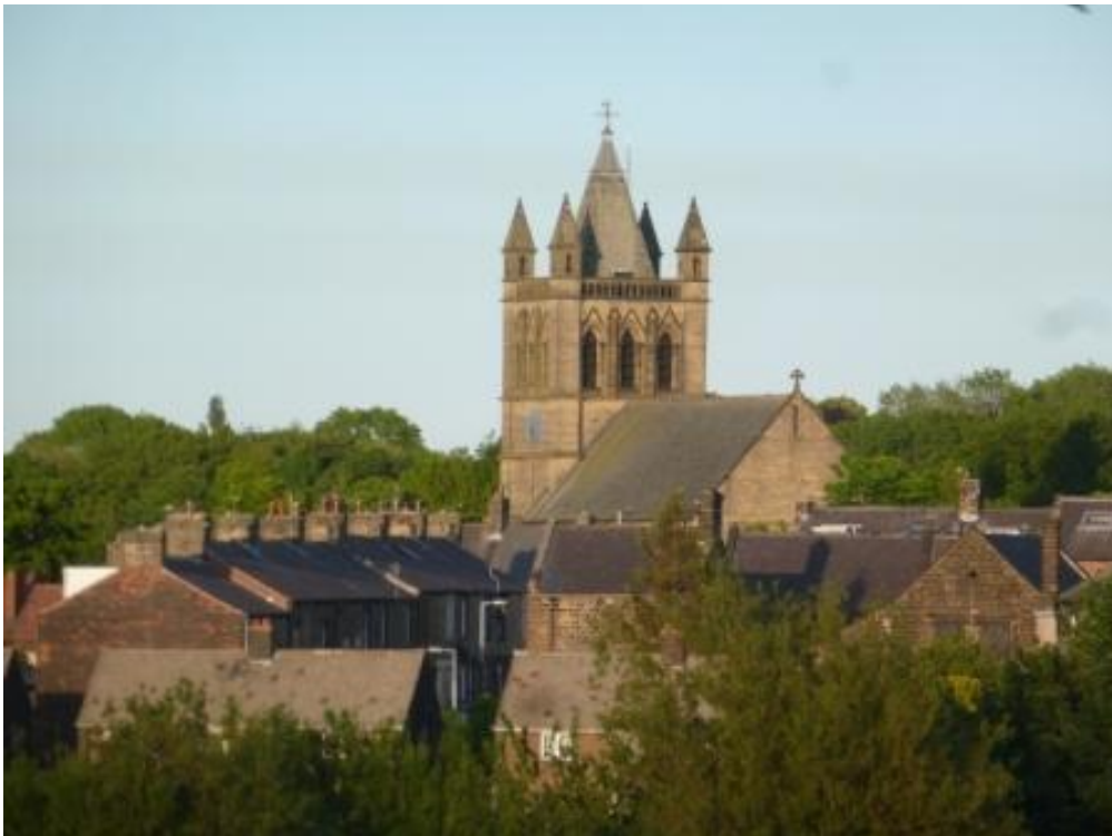
View from Locke Park
