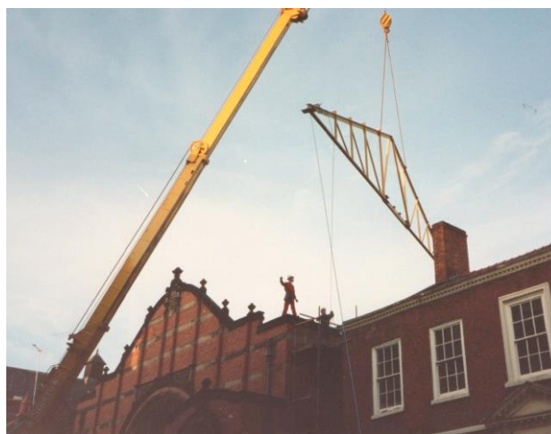
Fig. 43: New Roof Structure being Installed
