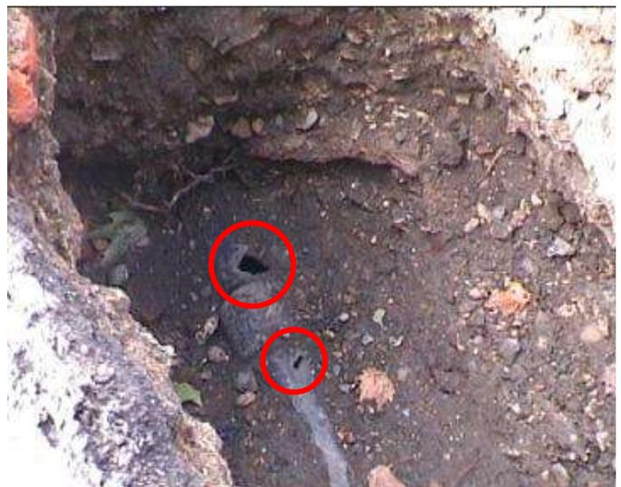
small section the pitch fibre had been perforated and almost certainly deformed or damaged elsewhere over a period which now well exceeds its useful maximum lifetime of 40 years or so.
