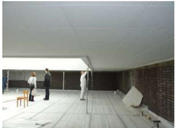
As the ceiling tiles were removed it was clear that there had been years of damp caused by water penetration through the failed upper flat roof asphalt and through leaking pitch fibre rainwater goods at that level.
