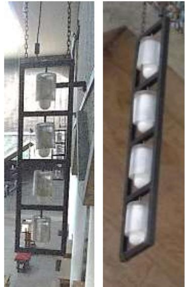
as the spotlights fail the bulbs cannot be replaced without installation of mid-height scaffolding. The perimeter lights simply do not illuminate the seating area and so as the spotlights continue to fail the seating area is seriously underlit, especially at night. The intention at the time of my retirement was to install low-energy long-life LED spotlights.
