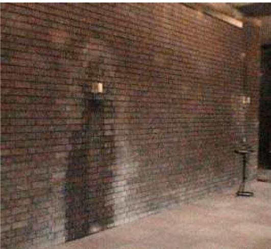
On May 24<sup>th</sup> 2001, after permission had been granted, another approach was tried out on the most heavily leaking downpipe on the north wall of the church (shown here).
