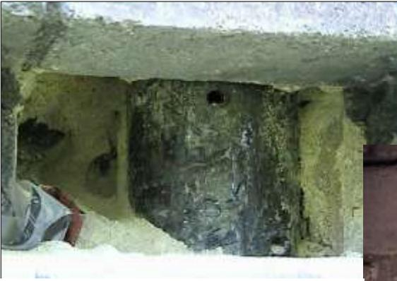
In these unique views the black pitch fibre downpipe can be seen emerging from the encasing mortar which holds it in place within the cavity. The solution adopted was to entirely encase the collar in (I think) a version of roofing felt and any standing water in the pipe would not then
