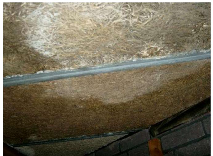
Because of the failure of the upper flat roof and leaking rainwater goods, clear signs of damp can be seen. Repairs to both have put a stop to this and damp areas have dried out.
