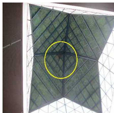
Figure 3. Location of wood wool ceiling panels which fell from the high level lantern in July 2013
