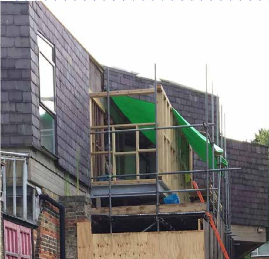
Work on the cantilevered extension to the church sanctuary has begun, and, as you will see from the photograph on the left taken on 31 August, the extension floor and framework is under construction. If all goes to plan we will have a fully disabled-accessible toilet and baby-changing facility and a new refreshment serving area by the beginning of December.
