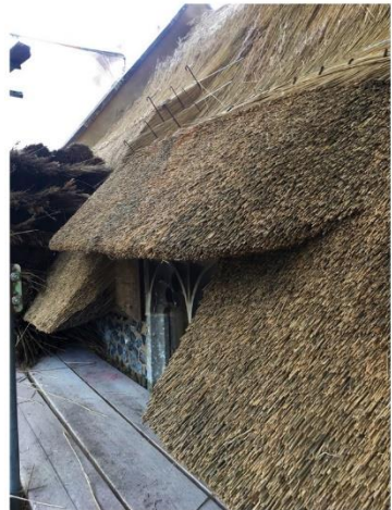
Progress on the rethatching of Beighton Church
