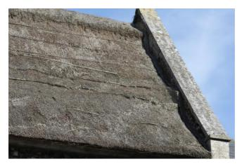
The nave roof thatch needs completely replacing and a number of the trusses and2 scissor-brace beams need repairing or possibly replacing.
