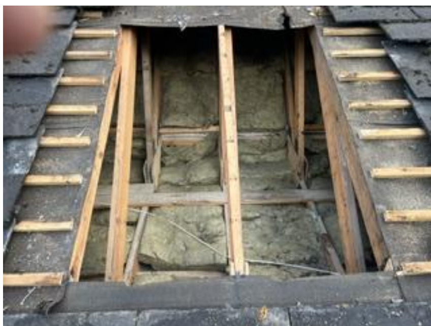
Not the prettiest view of the church – roof repairs in progress!
