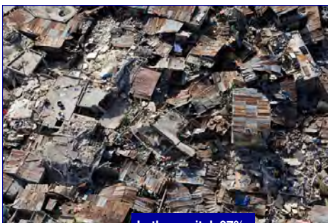
In the capital, 97% of the houses have collapsed
