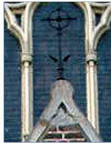
The west porch iron cross replaced the original stone cross
