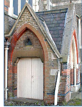
The west porch built in 1881
