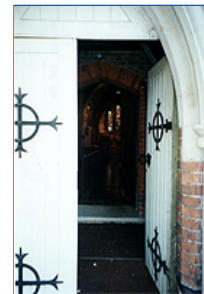
The old west porch doors
