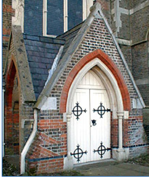
The west porch built in 1881
