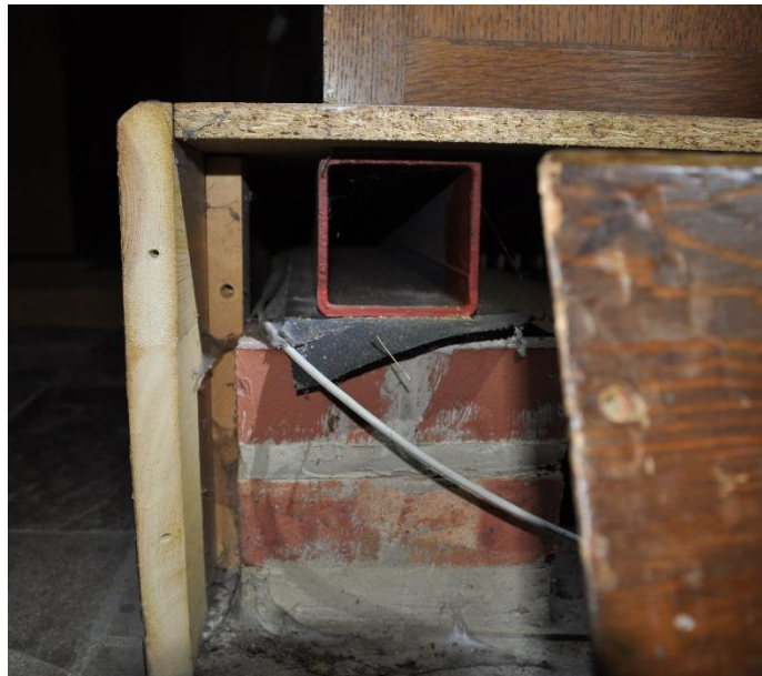
Figure 32 The western end of the organ platform with the western apron piece removed showing the brick pier and steel framing within. The oak board on the left-hand side would be moved in to tightly abut the steel box section.
