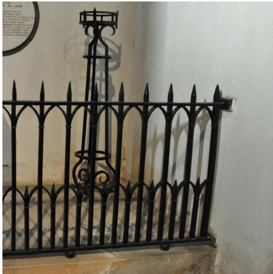
Figure 30 (Left) The Cowper sanctuary railings showing the projecting wall fixing. This was originally embedded in timber panelling.
