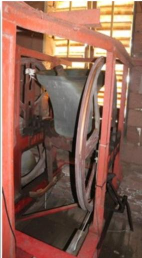
working parts that enable change-ringing to be done (the big timber rope wheels, bearings, clappers, rope guides, etc.) now need replacing or refurbishing.
