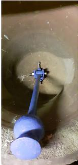
In April this year we asked advice from Whites of Appleton. They told us they could make a modified clapper bolt, fitted with an adjustable staple unit. In effect, this provides adjusters known as twiddle pins inside the crown of the bell, enabling the clapper bush to be moved to and fro. Their provisional estimate for this work was less than £1000 provided we removed the clapper from the bell and delivered it to their workshop in Appleton, near Oxford.
