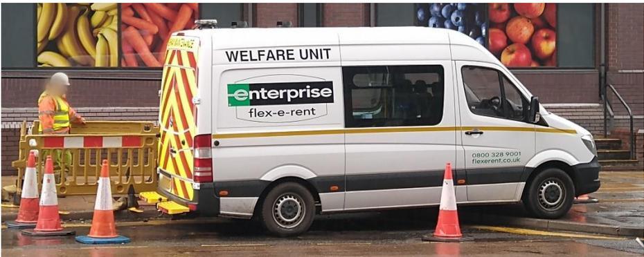
*CDM in action: The worker has access to welfare facilities in the van. The site is clearly defined and measures have been taken to protect the public from the site (a hole in the pavement surrounded by fencing) and the worker is protected from traffic by the road cones.*
