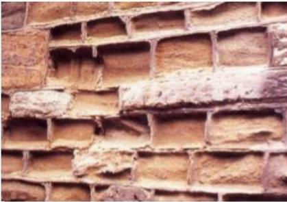
*Hard cement pointing has caused the soft stone to decay*
