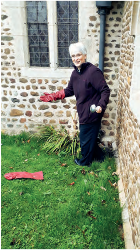
Annette clearing the drains at Little Paxton during a Faith in Maintenance workshop
