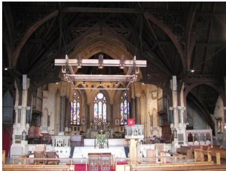
Central sanctuary area
